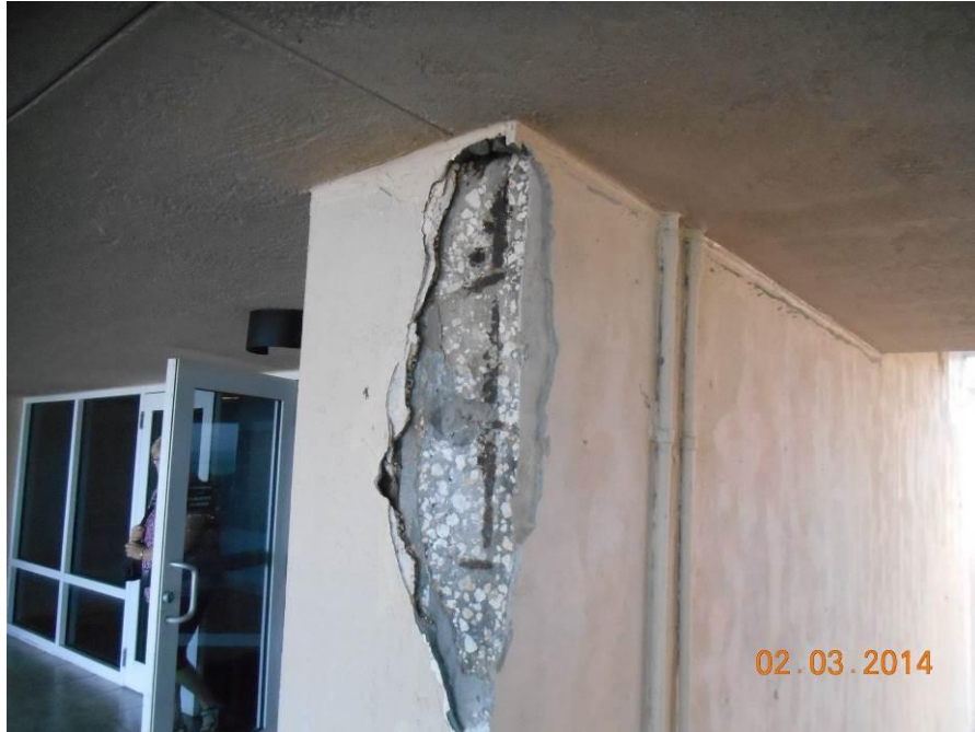
Concrete spalls requiring excavation on the east parking garage shearwalls.
