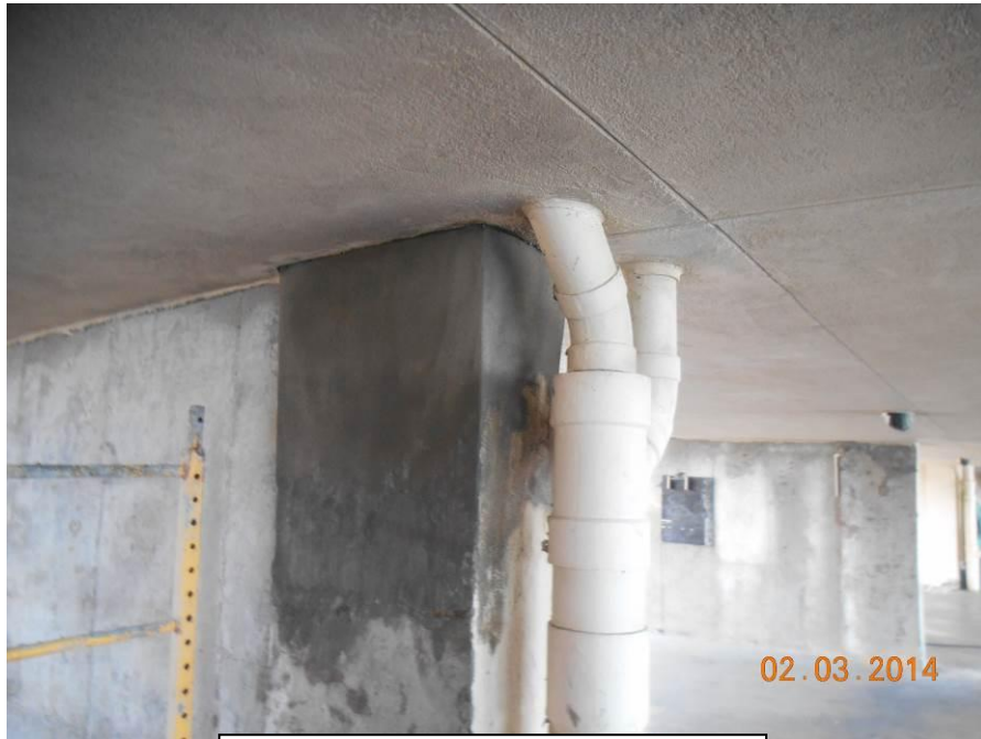
Patching mortar repair finished on east parking garage bay shearwall.
