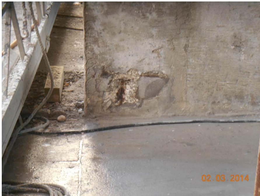
Concrete spalls requiring excavation on the east parking garage shearwalls.
