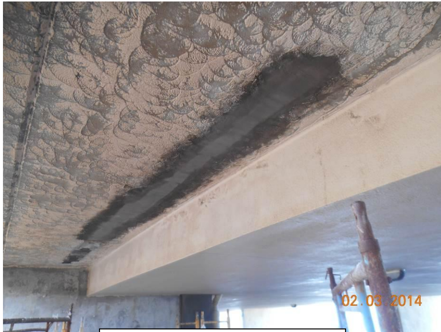
Patching mortar repair completed on east parking garage hollow-core ceiling panel.
